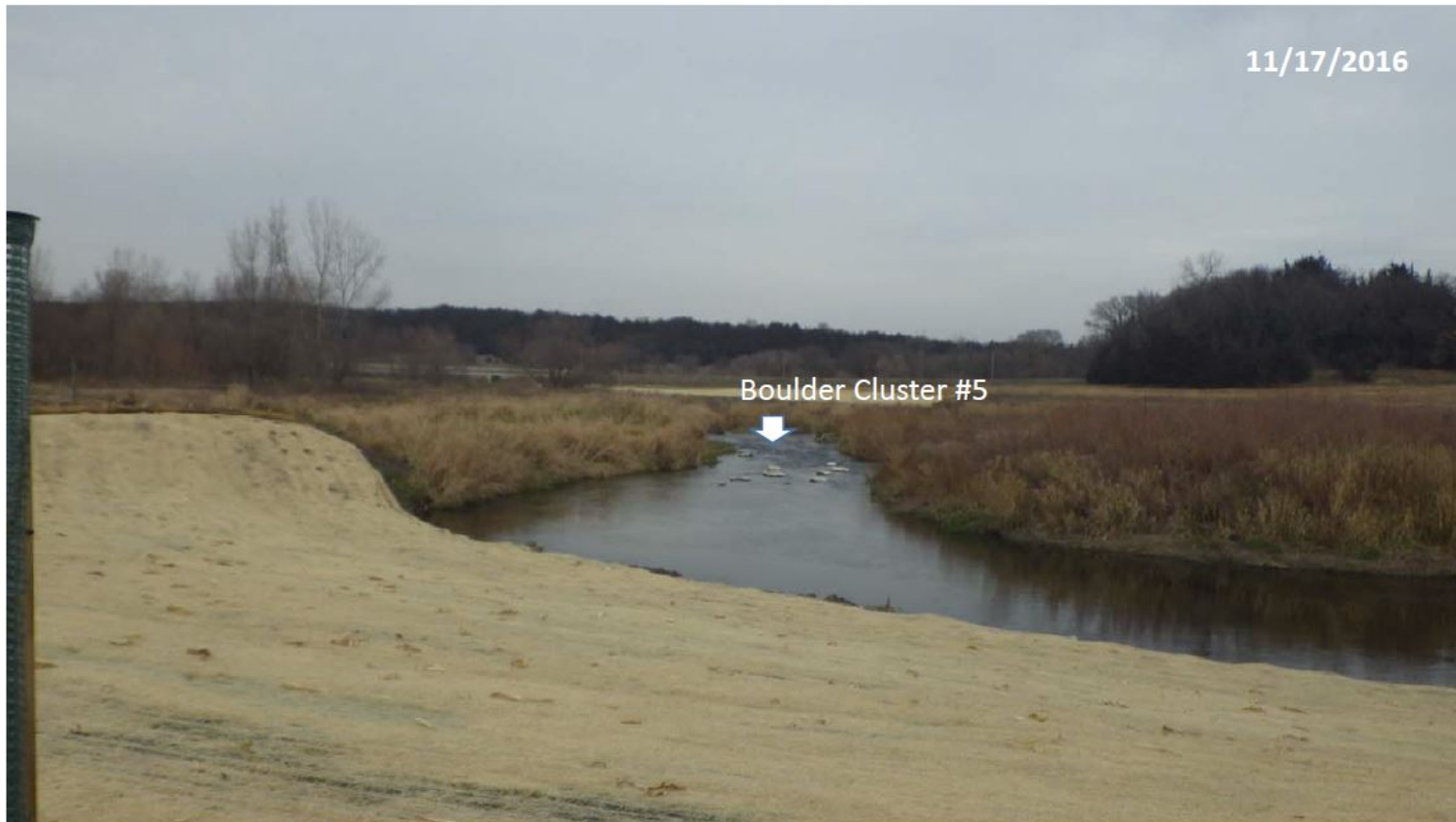
Boulder Cluster #5 – Looking North (Upstream)
